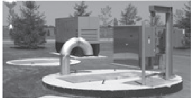
Lift Stations-New and Retro-fit Upgrades
